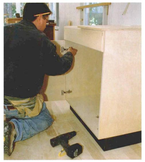
**Pop on the doors.** If holes have been drilled correctly, hinges installed on cabinet doors should snap easily into place on the base plates. These hinges allow the author to fine-tune the fit of the door.
