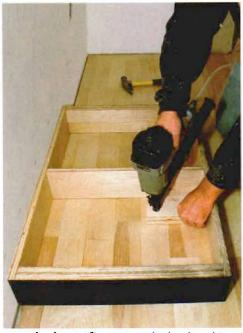
Set the bases first. To make leveling them easier, the author installs the bases separately from the cabinets. With the bases secured, he then sets the cabinet boxes in place and screws them to the wall.
